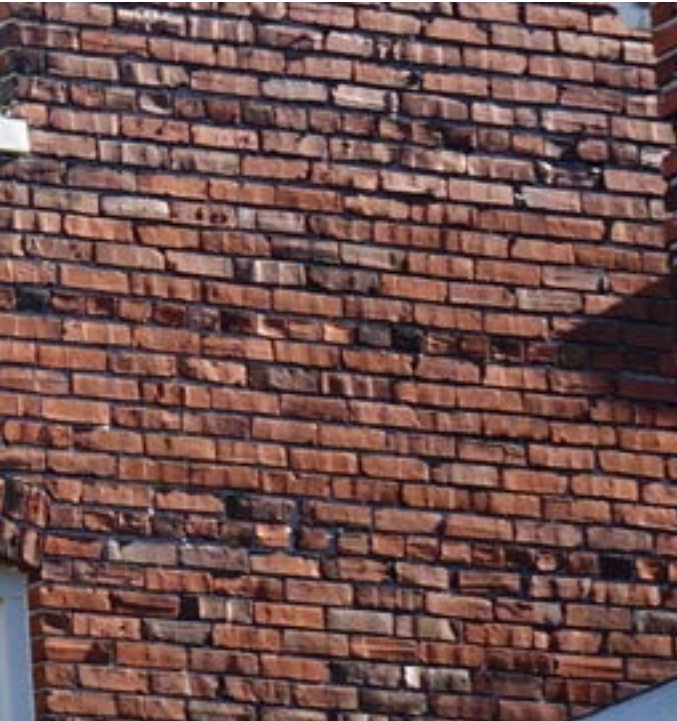
Common bond is a pattern of one row of brick headers, an odd number of stretcher rows, and another row of brick headers. Staff, 11/6/2025.
