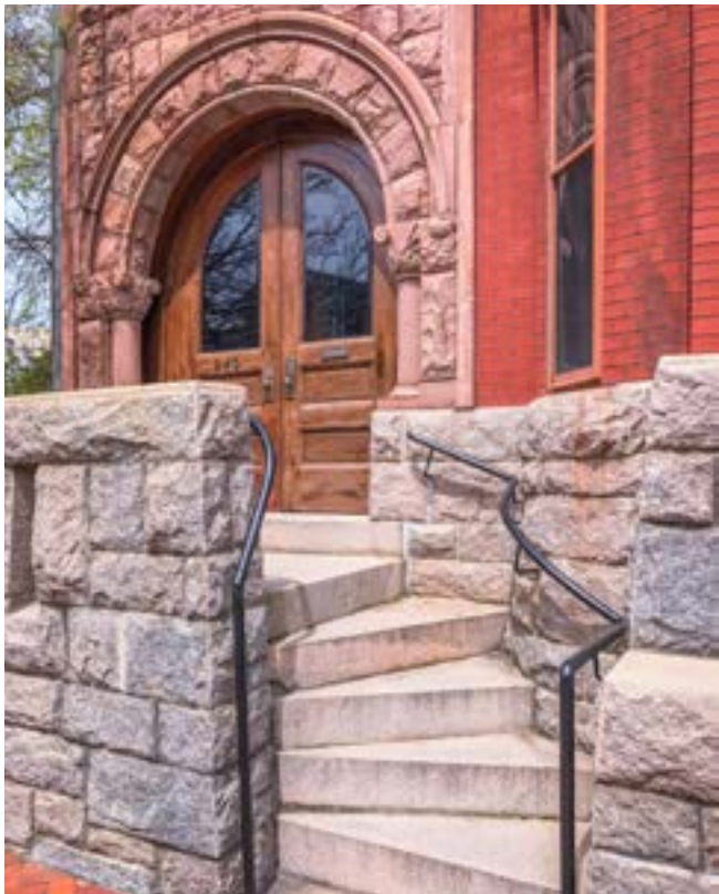
Different masonry materials are sometimes used together for a variety of wall textures and as accent features. This building has brick, dressed stone, and rough cut stone, which are major character-defining features. Suping Li, 2017.
