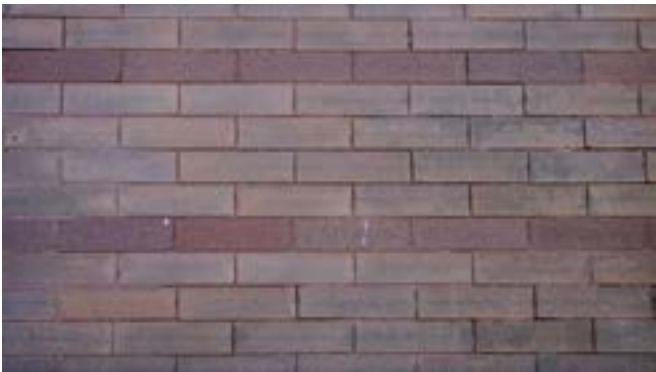
Stretcher bond, also known as running bond, alternates stretcher rows. Staff, 11/6/2025.
