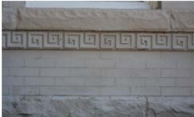
Carved masonry defines the wall beneath a stone sill. 11/6/2025
