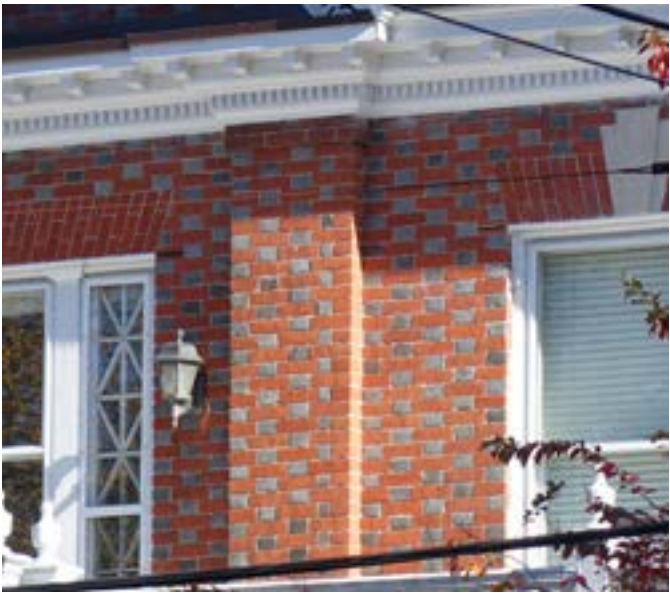
Flemish bond is one of the most ornate bond patterns and is sometimes only found on the primary elevation of a building. Flemish bond is made by alternating brick headers and stretchers in each row. Glazed brick or differently color brick are often used. Staff, 11/6/2025.
